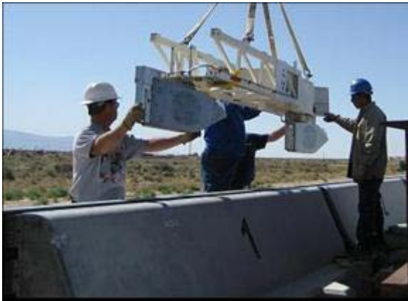
Figure 9. Sled/magnet shown being installed in guideway
