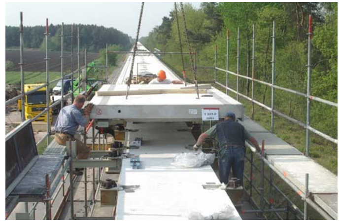
Figure 5. Track of Type III, Züblin design (Source: Ed.Züblin)
