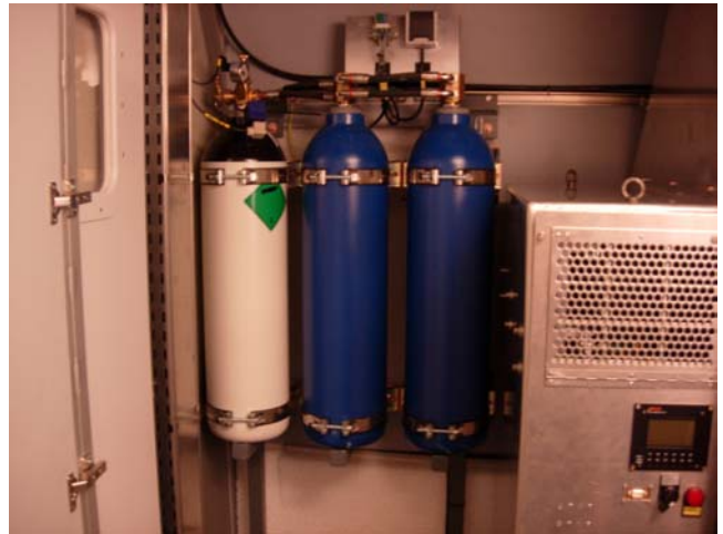
Figure 10. TR09 fire fighting system, pressure bottles
